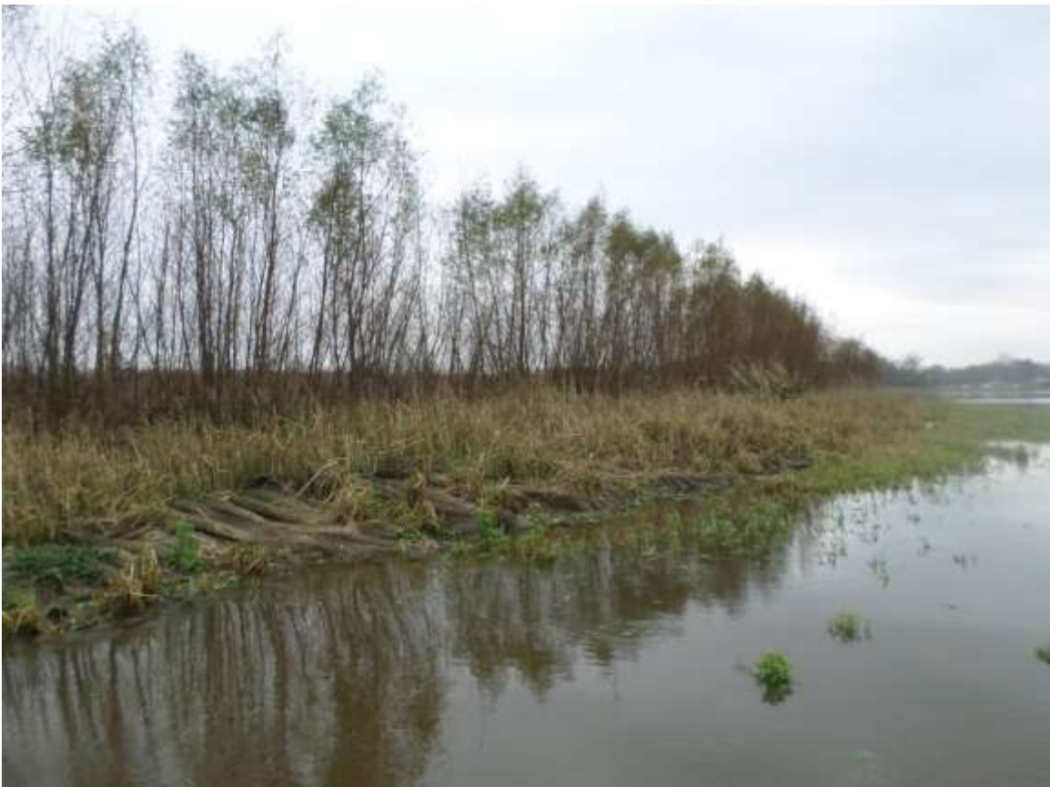
Pic #10: NW corner of the island looking along the shoreline protection mats – much vegetation
