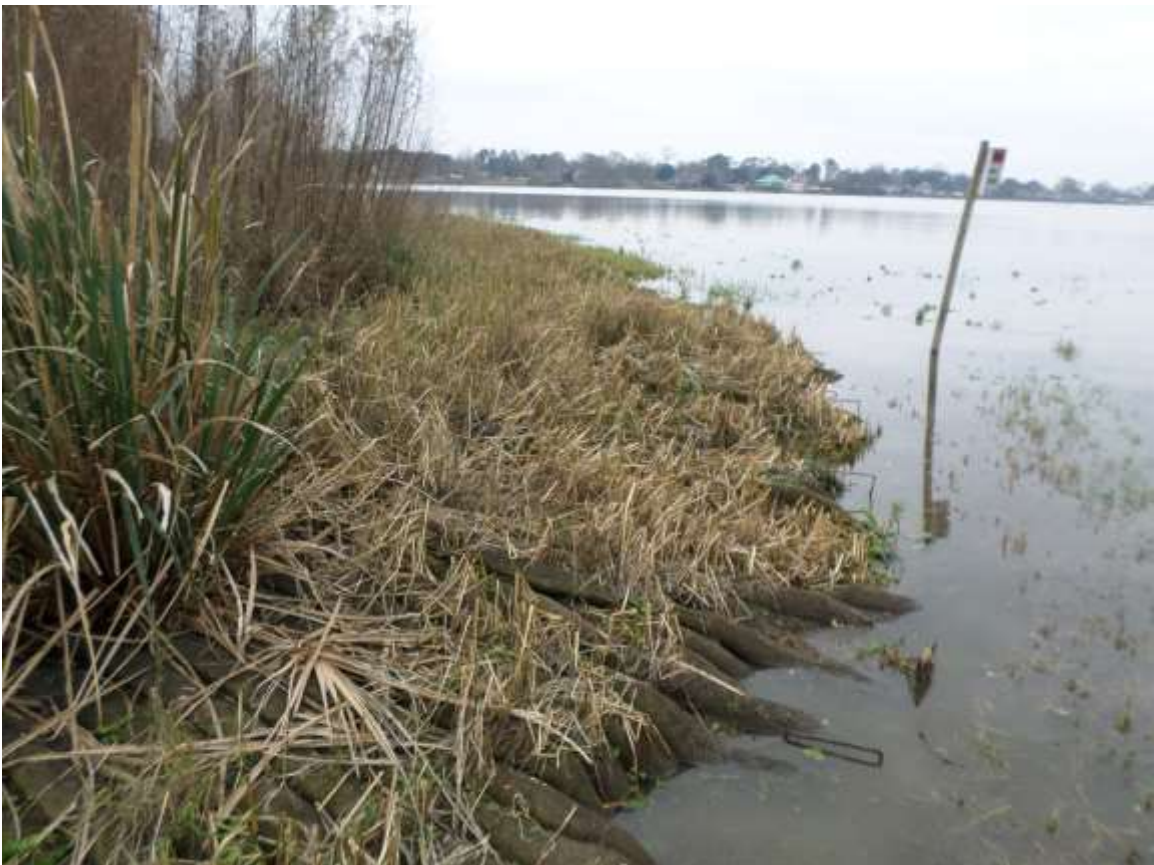
Pic #8: NW corner of the island looking at the shoreline protection mats – much vegetation
