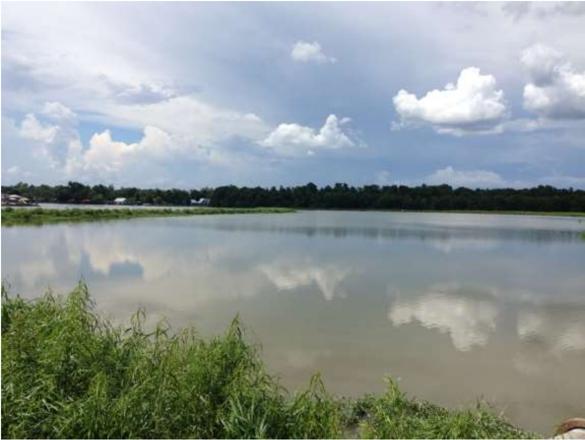
June 11, 2015 – View of the front (west) levee and inside of the island
