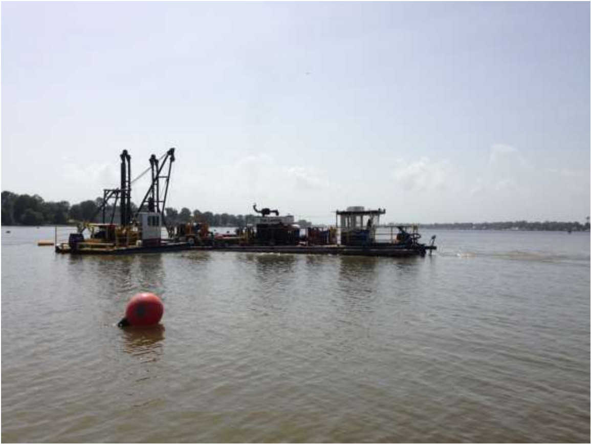
Dredge in full operation
