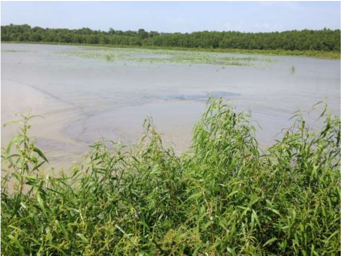
Dredge material being discharge inside the island's berm
