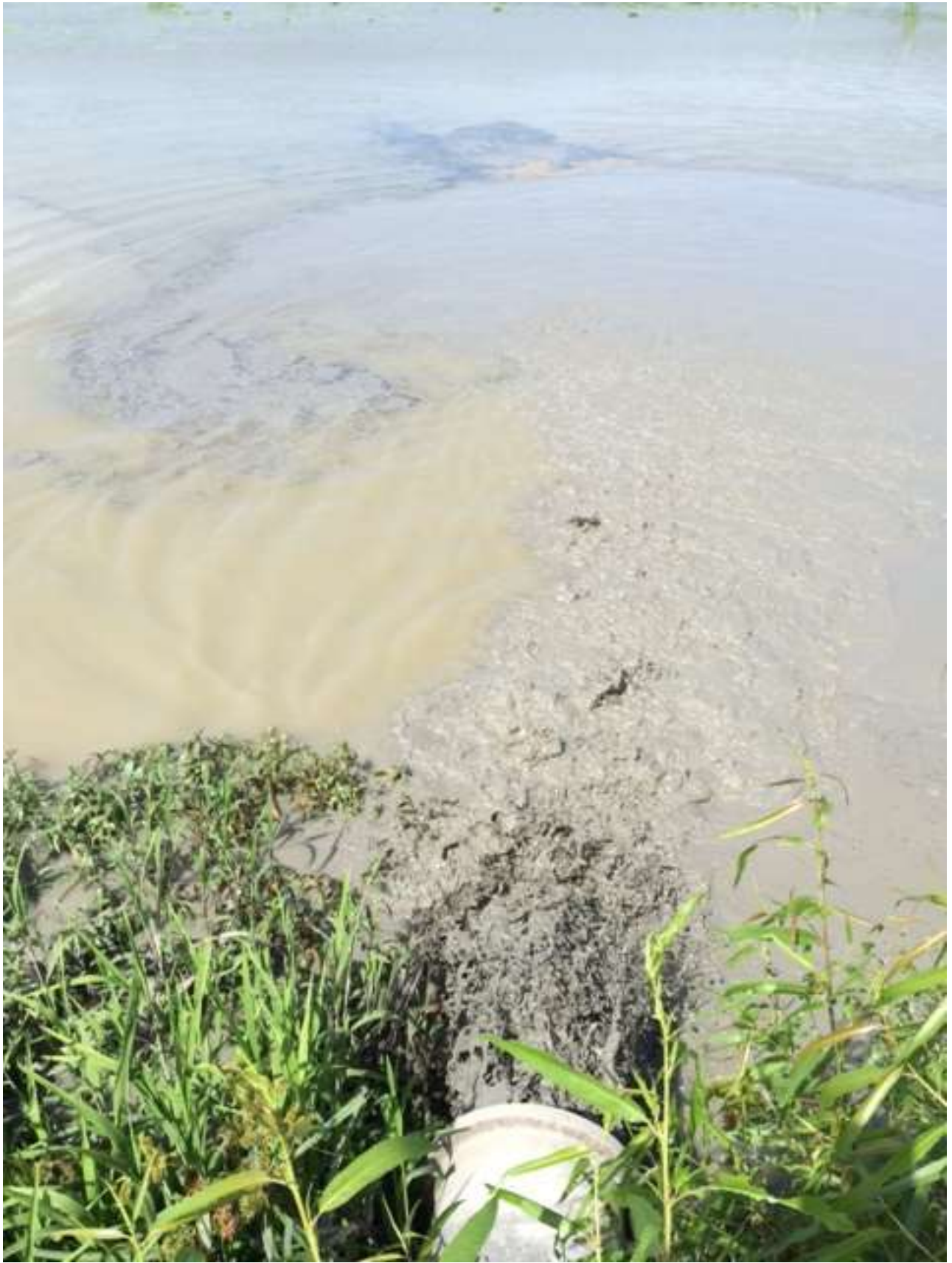
Dredge material being discharge inside the island's berm
