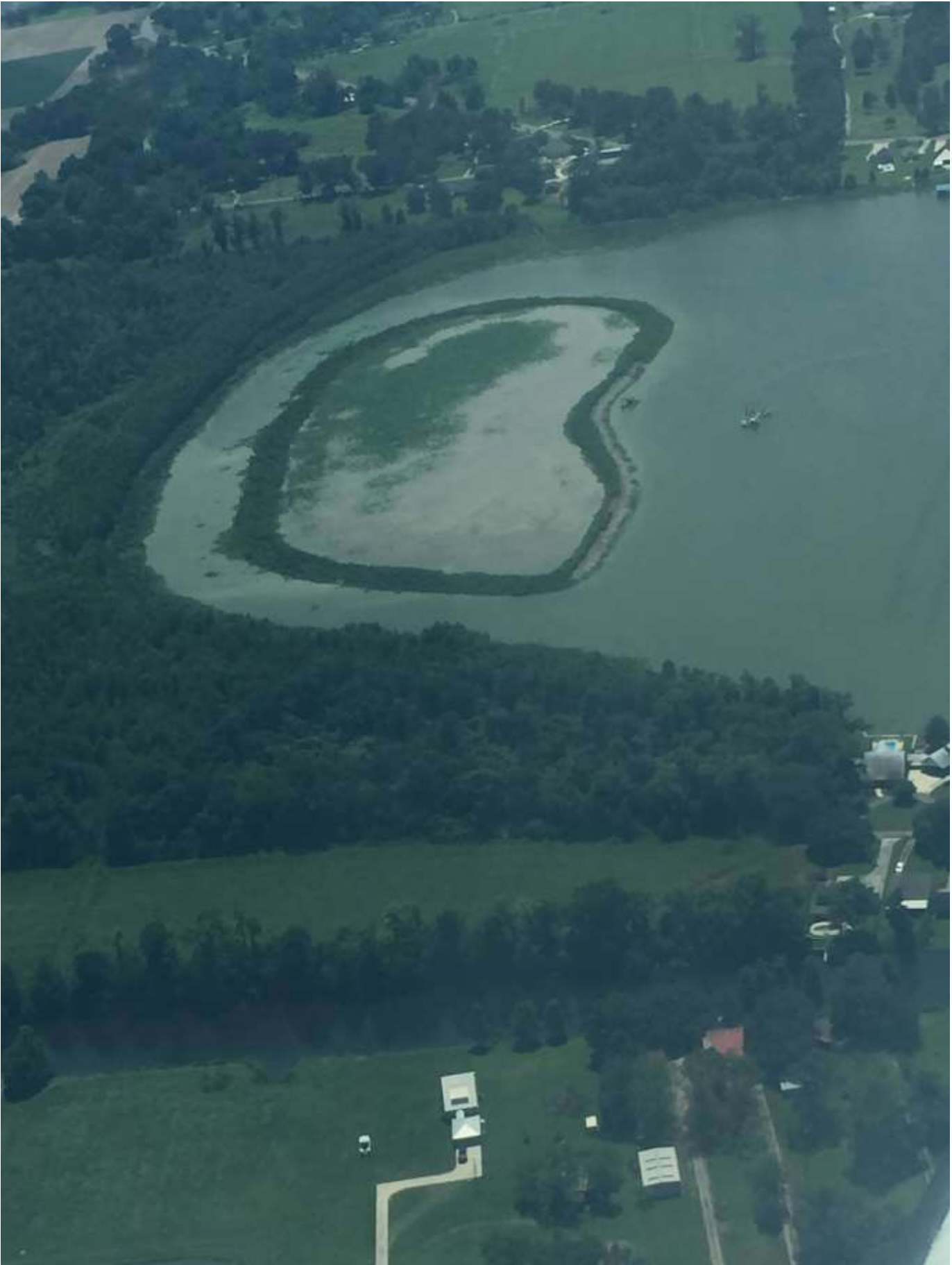
Photograph taken 8/13/15 courtesy of RLB Contracting, Inc.
