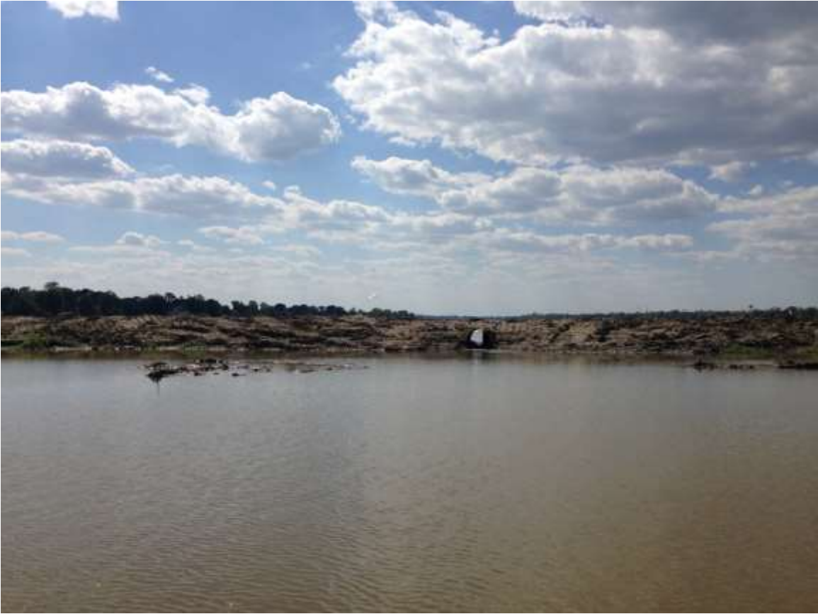
Easternmost outfall in the island's berm (4/30/15)
